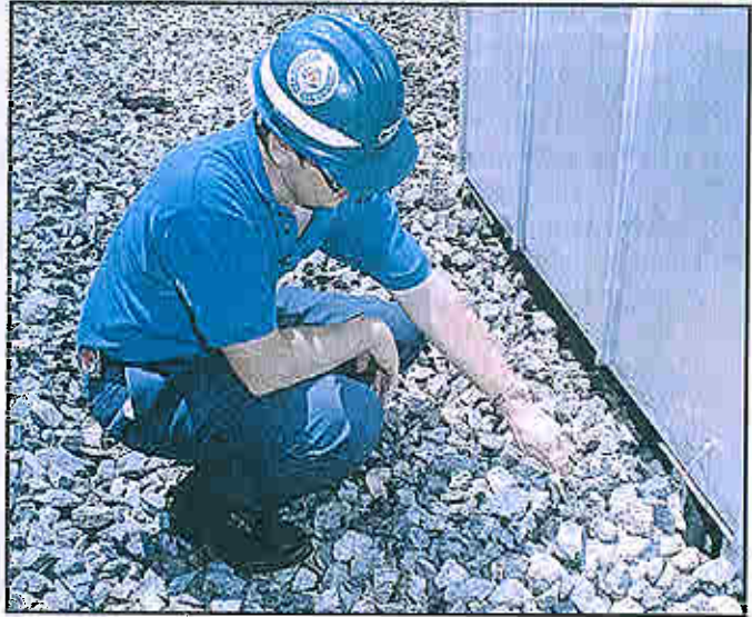
Figure 6-3: Inspecting the ground rods and connections
