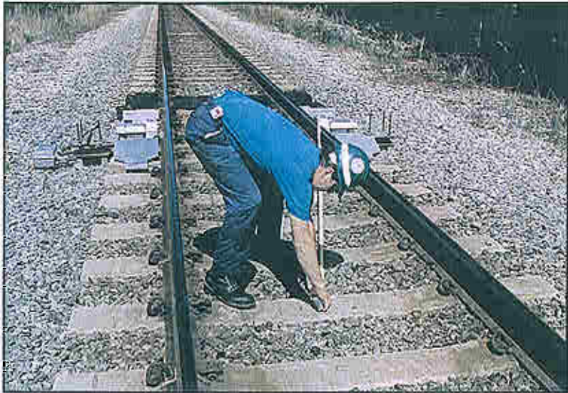
Figure 6-11: Maintainer using triangulation procedure
