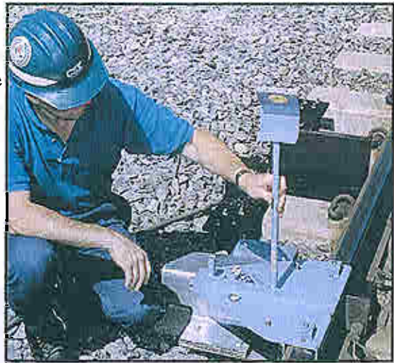
Figure 6-13: Alignment fixture attached to a rail
