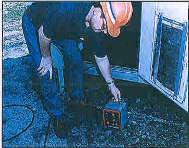
Figure 8-9: Placing the function simulator outside in the shade
