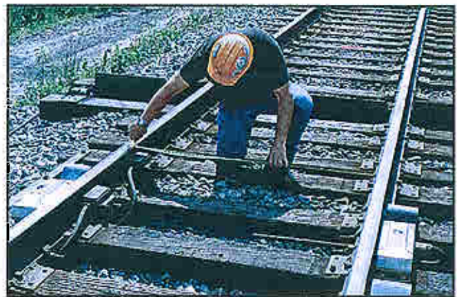
Figure 8-20: Measuring the track gauge
