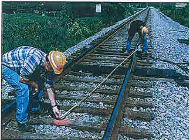
Figure 8-12: Maintainers using a triangulation method
