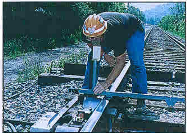
Figure 8-15: Looking through the peep hole to check the alignment
