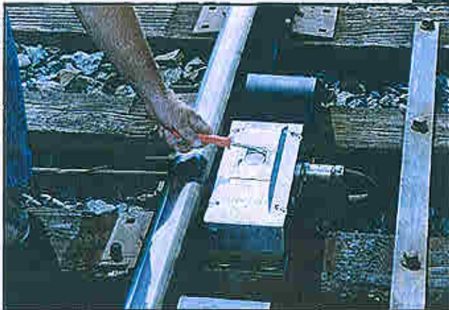
Figure 8-7: Using a soldering iron to fire hot boxes from the rail
