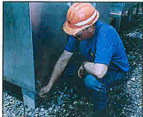
Figure 7-2: Checking the ground rods
