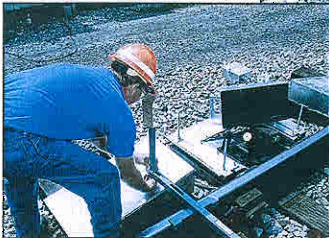
Figure 7-16: Looking through the peep hole to check the alignment
