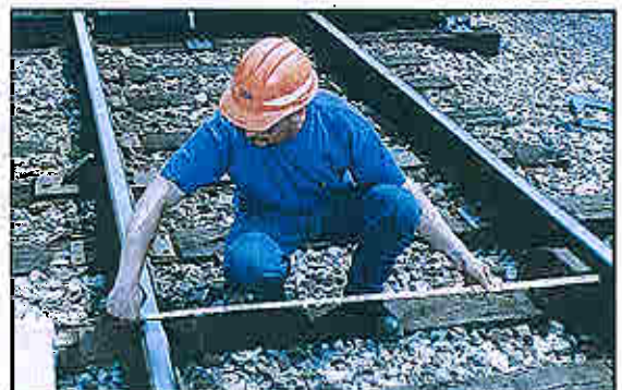
Figure 7-18: Measuring the track gauge
