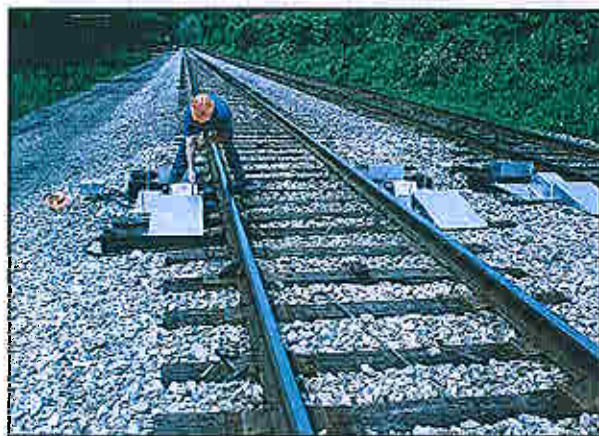
Figure 7-12: Maintainer using a triangulation method 9/30/95
