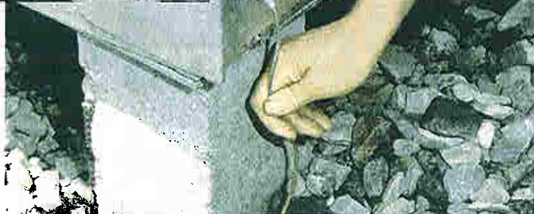
Figure 12-3 Inspecting ground rod.
