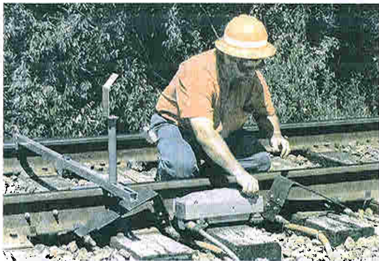
Figure 12-15 Replacing scanner covers.
