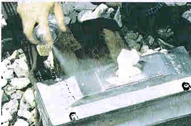
Figure 12-4 Spray painting scanner cover.
