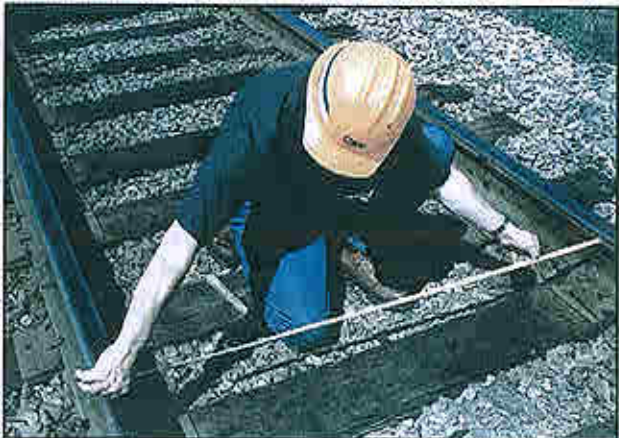
Figure 11-20: A maintainer observing the surface of the track as a train passes and checking track gauge.
