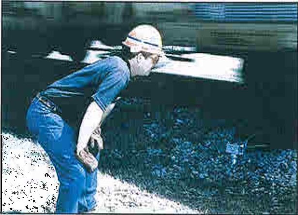
Figure 11-20: A maintainer observing the surface of the track as a train passes and checking track gauge.
