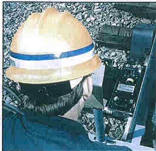
Figure 11-15: Looking through the peep hole to check the alignment
