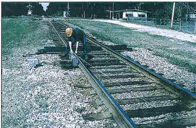
Figure 11-12: A maintainer using triangulation to ensure squaring of the scanners
