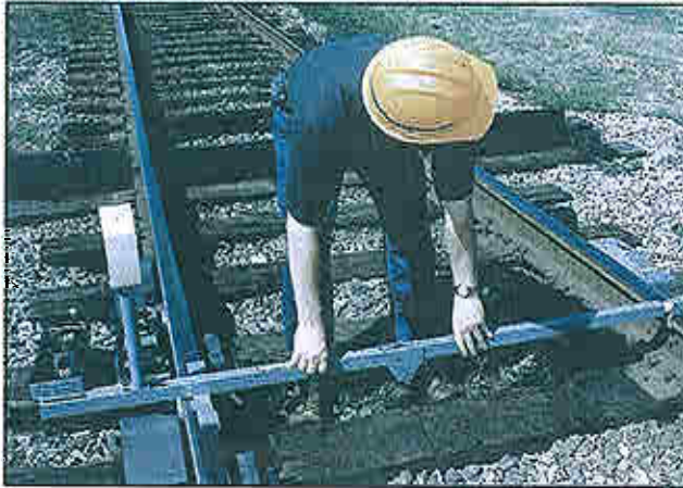
Figure 11-14: Setting up the alignment fixture and lens cap
