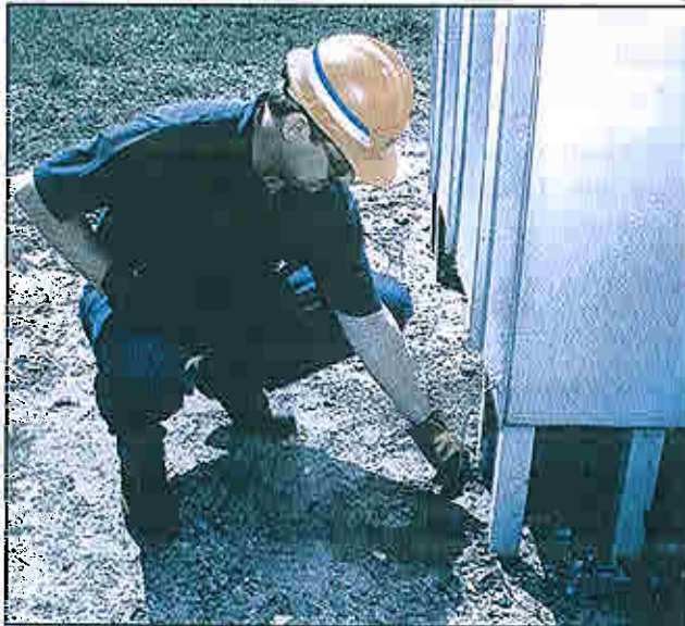
Figure 11-3: Inspecting the ground rods and connections
